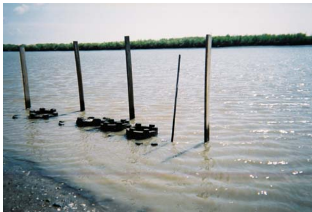
Figure 3.6: Emplacement in estuarine waters in southern Louisiana shows an intertidal placement (rings are slightly emerged at low tide, and may be submerged during high water).
